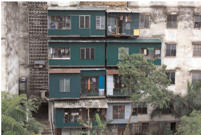
Figure 5: Residential redesigns and expansions in Quang Trung, 2011
